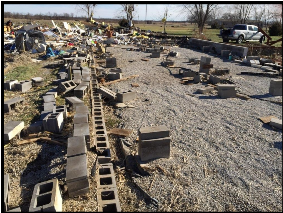
Mobile home destroyed by EF-1 tornado Dec 4, 2017
