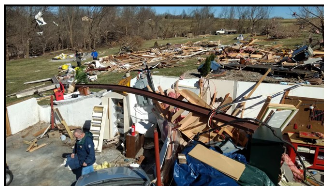
Destroyed house near Smithville Lake
